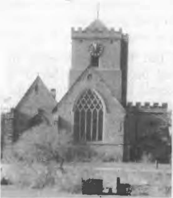
6 Shifnal Parish Church
